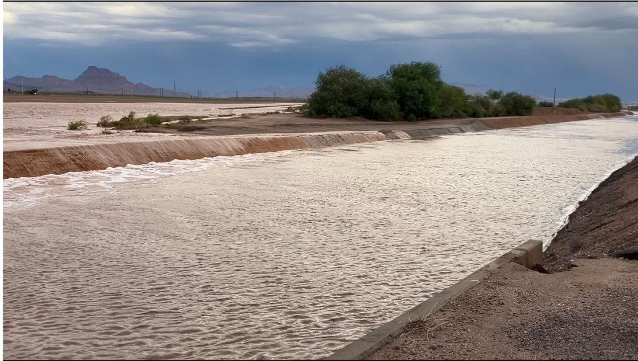
The Arizona Canal at Alma School Road 9/26/2025
