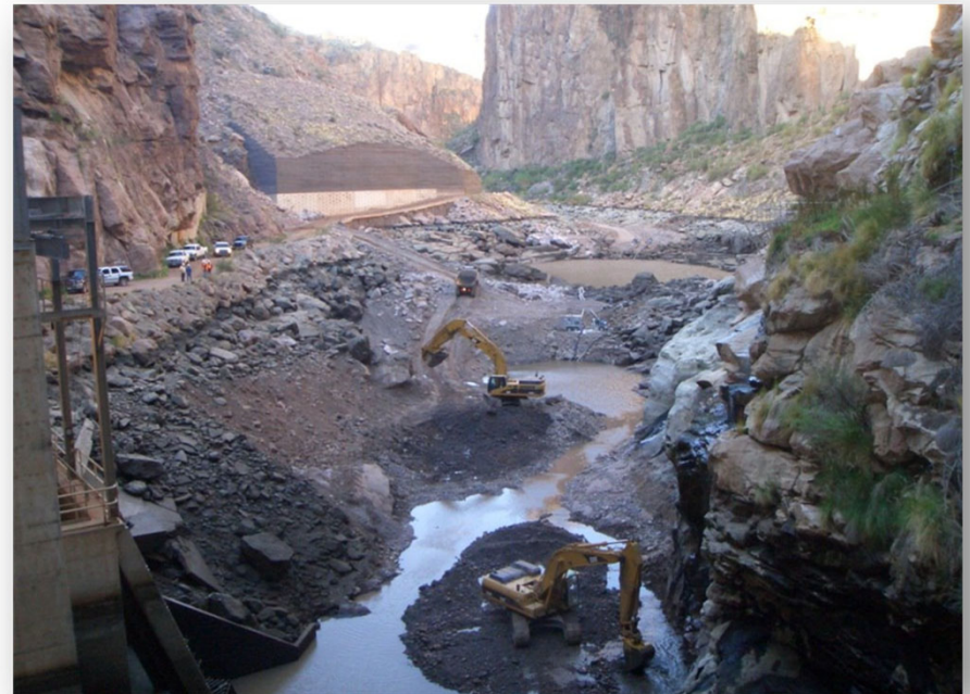
HMD Tailrace and Plunge Pool Work in 2007
