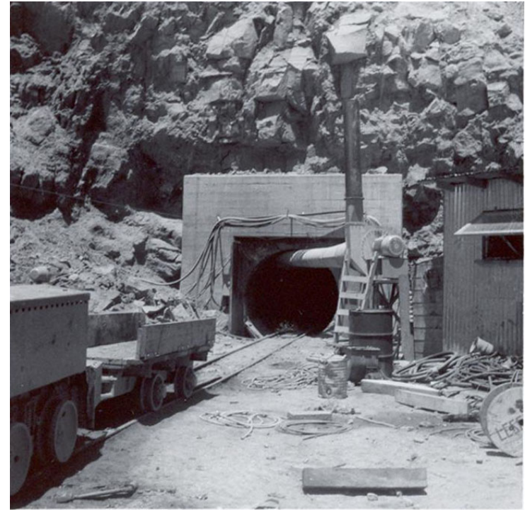
Construction of pumping system inlet tunnel (1965)
