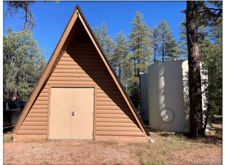
Verde Glen DWID – Pumphouse & Storage Tanks
