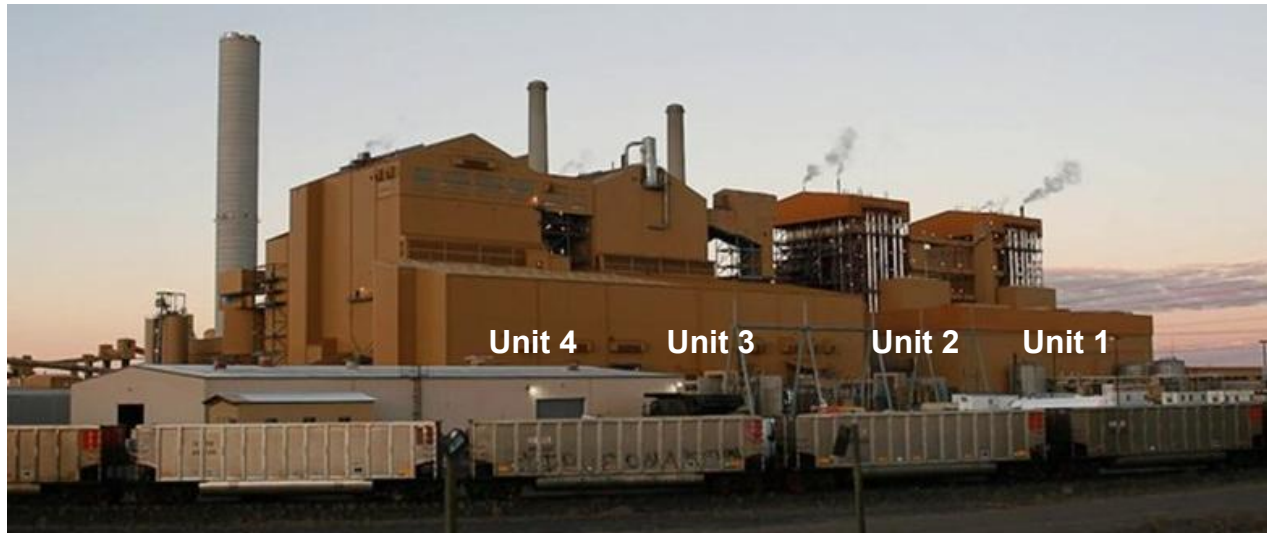
Figure 5. View of Existing Facility from the Southwest
