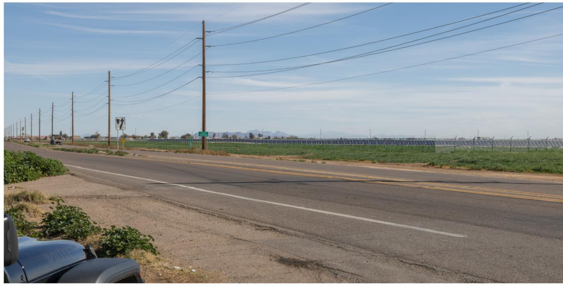
North Fuqua Road & State Route 84 – Looking Southwest
