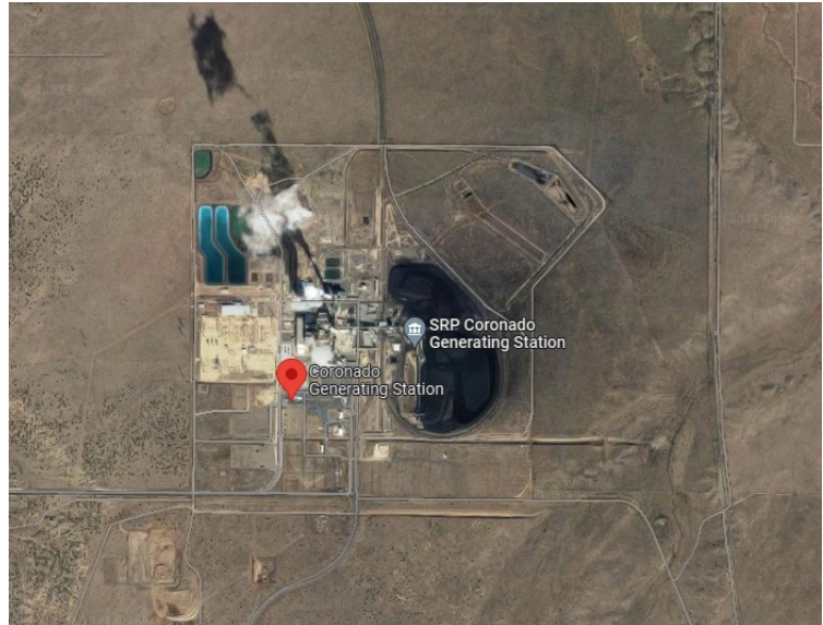
Figure 2A. Coronado Generating Station is in Apache County six miles northeast of St. Johns, Arizona.
