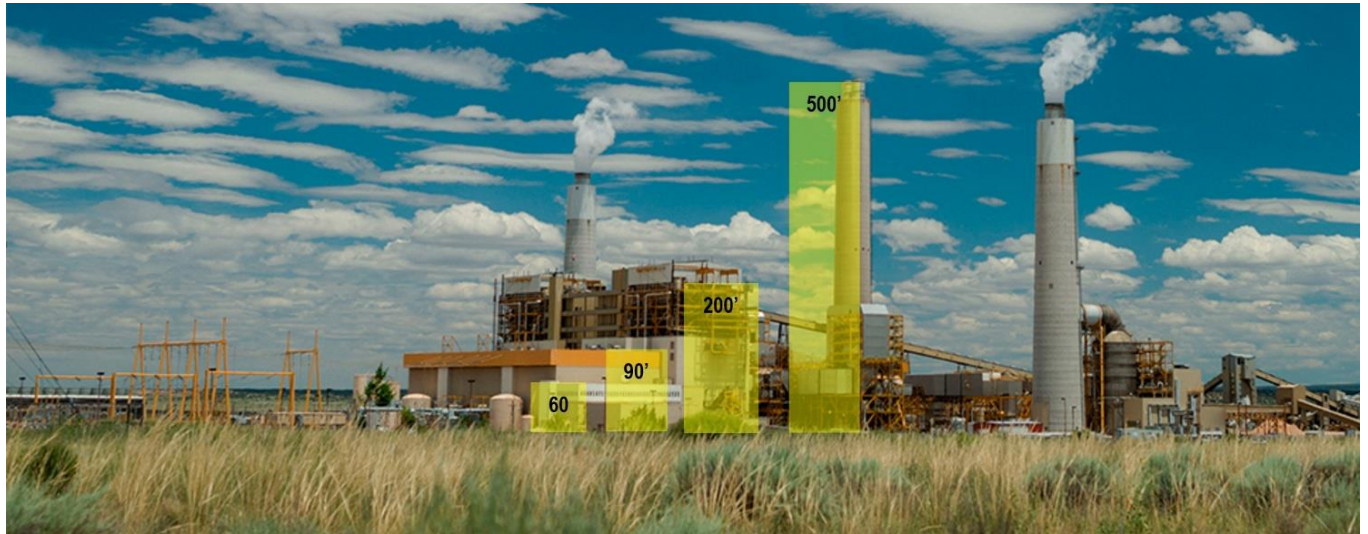
Figure 8. Photo & Scale of Existing CGS Facilities
