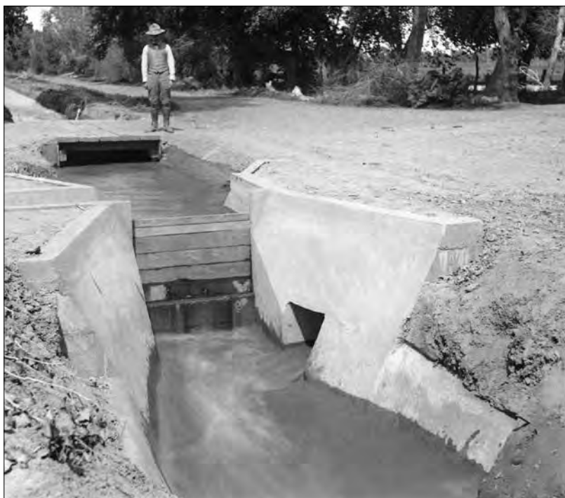
Zanjeros opened and closed gates like this one, circa 1900s, in order to deliver water.
