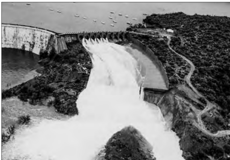
Stewart Mountain Dam with spillway gates wide open to release floodwaters of the Salt River, 1978
