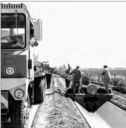
Slipform installation, 1968
