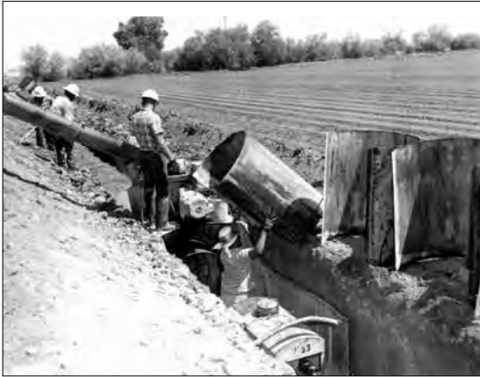
Cast-in-place concrete pipe installation, 1963
