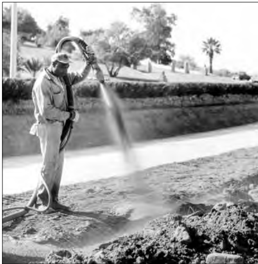
Gunite application on the Arizona Canal, 1967
