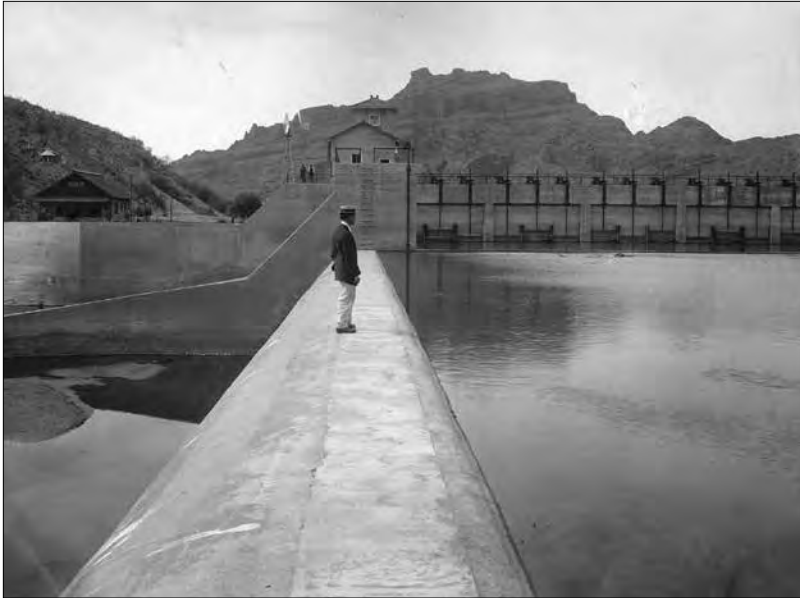
Granite Reef Diversion Dam and westside intake gates, 1911
