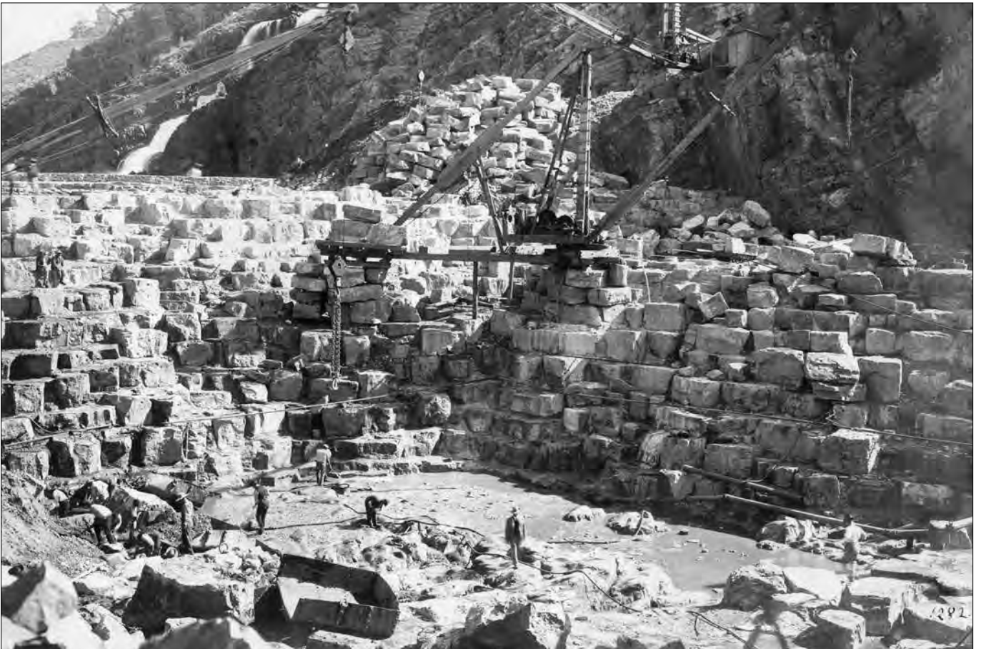
Top left: Preparing the foundation of Roosevelt Dam, laborers excavating down to bedrock, 1906
