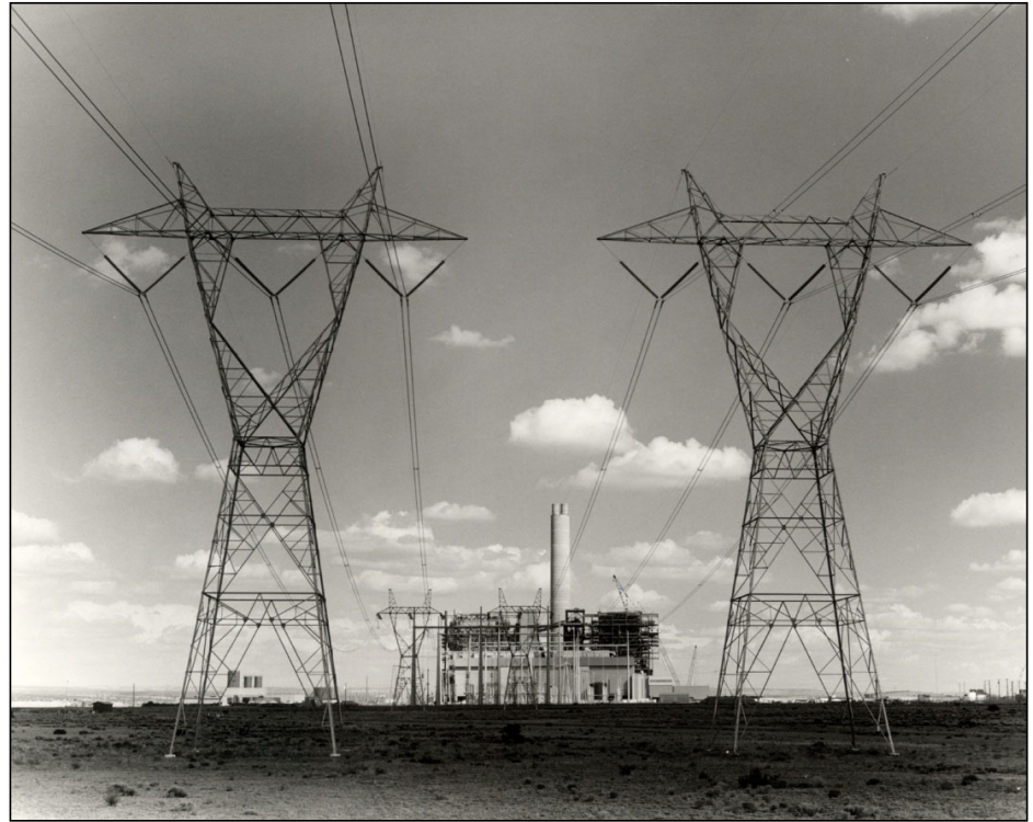
Coronado Generating Station, c 1980s
