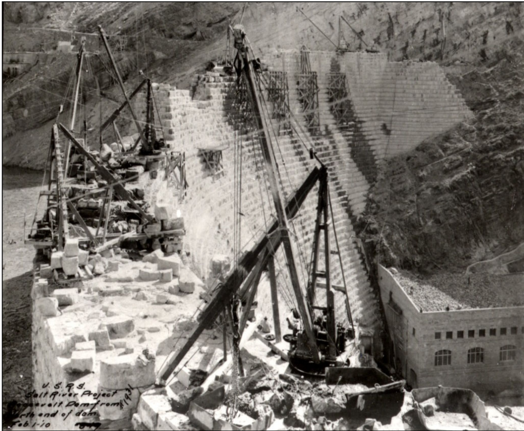
Roosevelt Dam construction, stiff legged derrick, 1910
