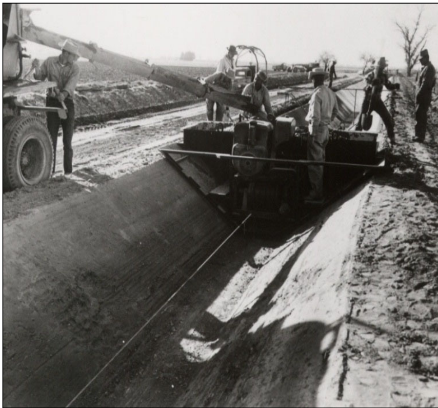
Slipforming lateral, c. 1960
