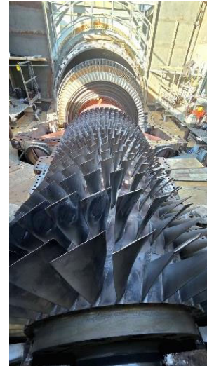
Gas turbine compressor
