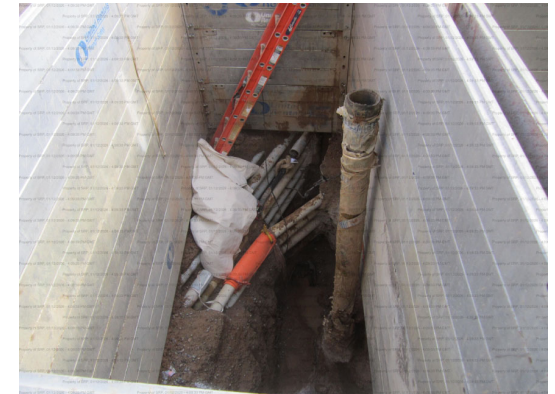
Blowdown line repair (underground)
