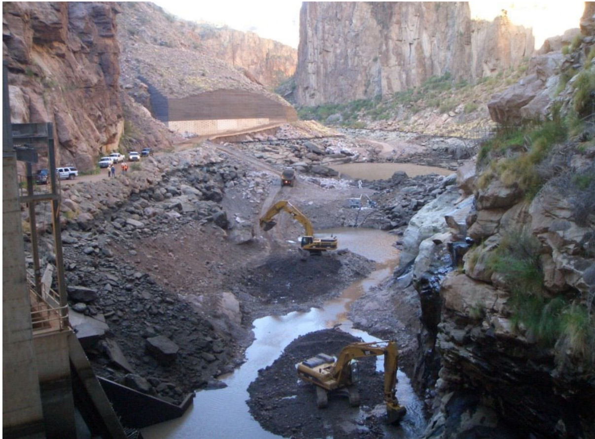
HMD Tailrace and Plunge Pool Work in 2007
