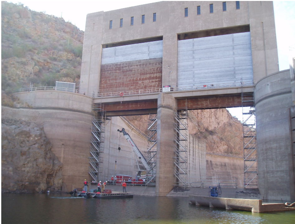
Gate maintenance being performed during the last Canyon Lake drawdown in 2007.
