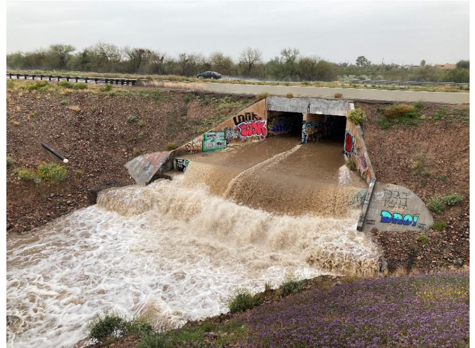
Evergreen Drain Box Culvert Under Beeline Highway
