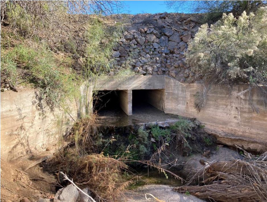
Box Culvert Under South Canal
