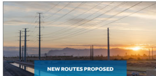
New transmission lines and substation
