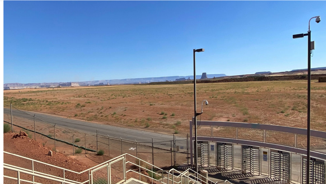
After the Decommissioning
