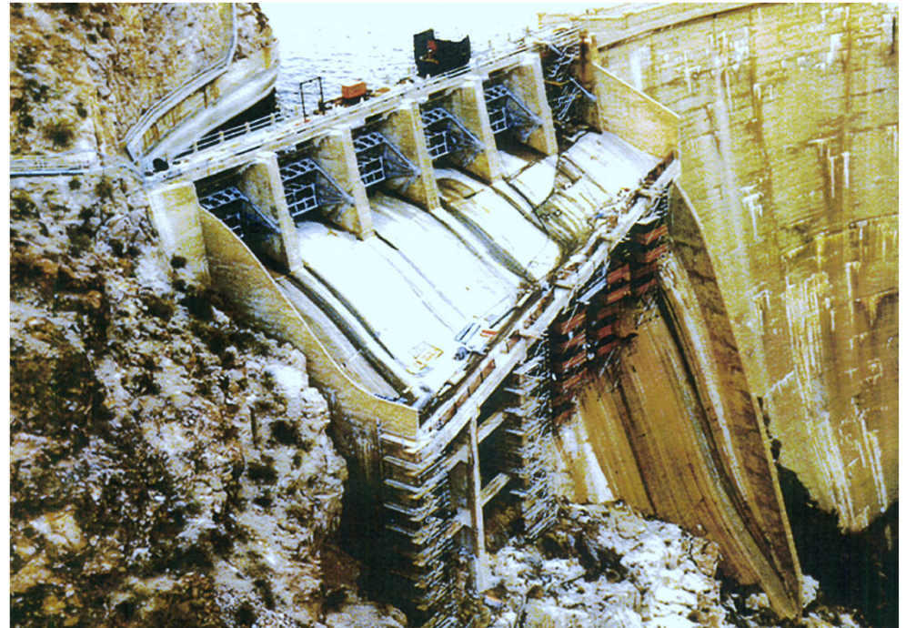
Horse Mesa Left and Right Spillways being repaired, with extensive scaffolding and equipment visible
