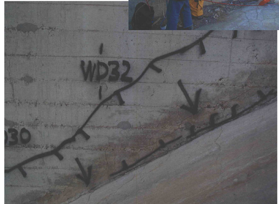
Visual inspection and sounding at Horse Mesa in 1999
