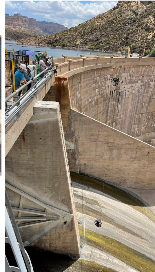
Sounding being performed on Horse Mesa Right Spillway in July 2022
