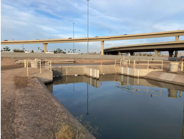
Western Canal Culverts East of I-10
