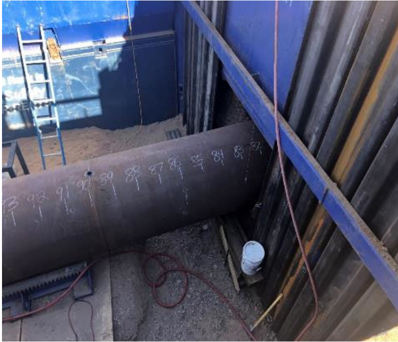
Steel Casing Pipe
