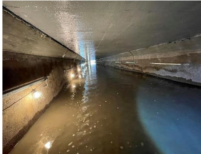
Finished Culvert Improvements
