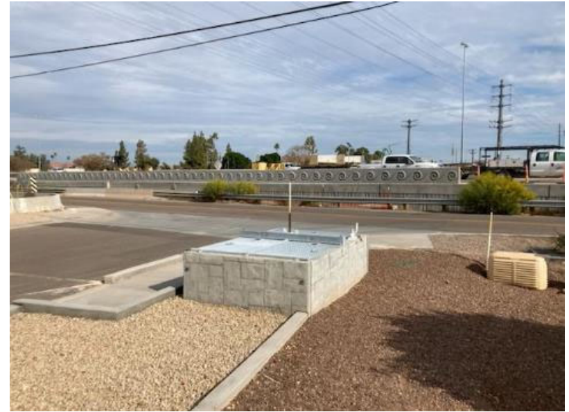
Irrigation Delivery Structure
