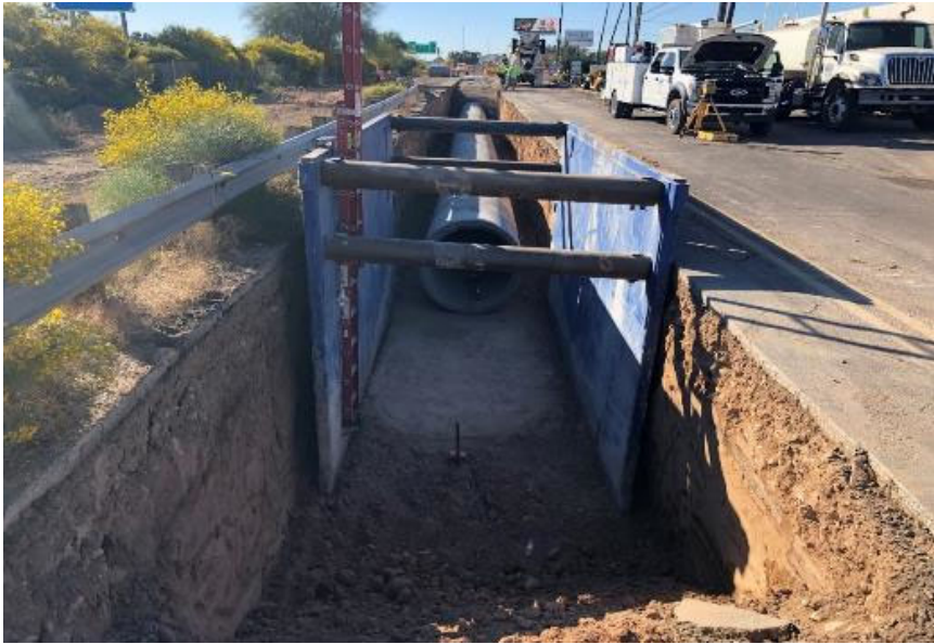
Irrigation Pipe Installation
