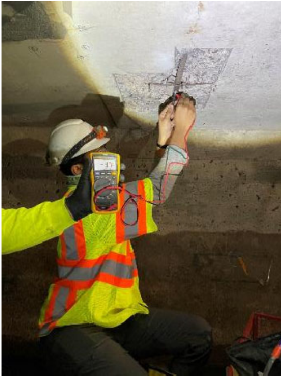
Cathodic Protection Work
