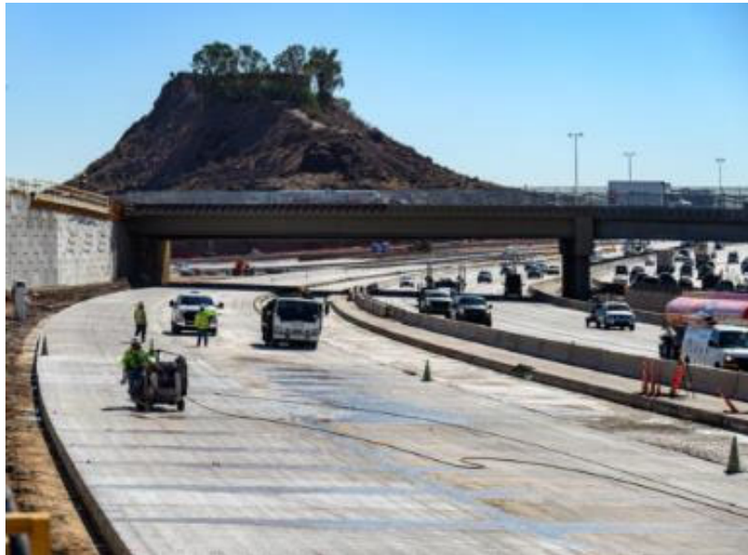
Interstate 10 Widening Near SR 143
