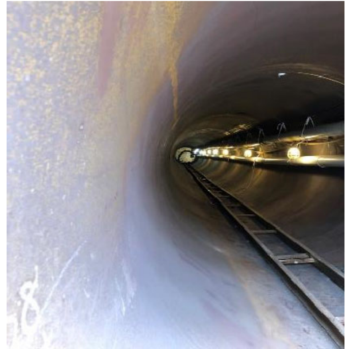
Inside of Steel Casing Pipe
