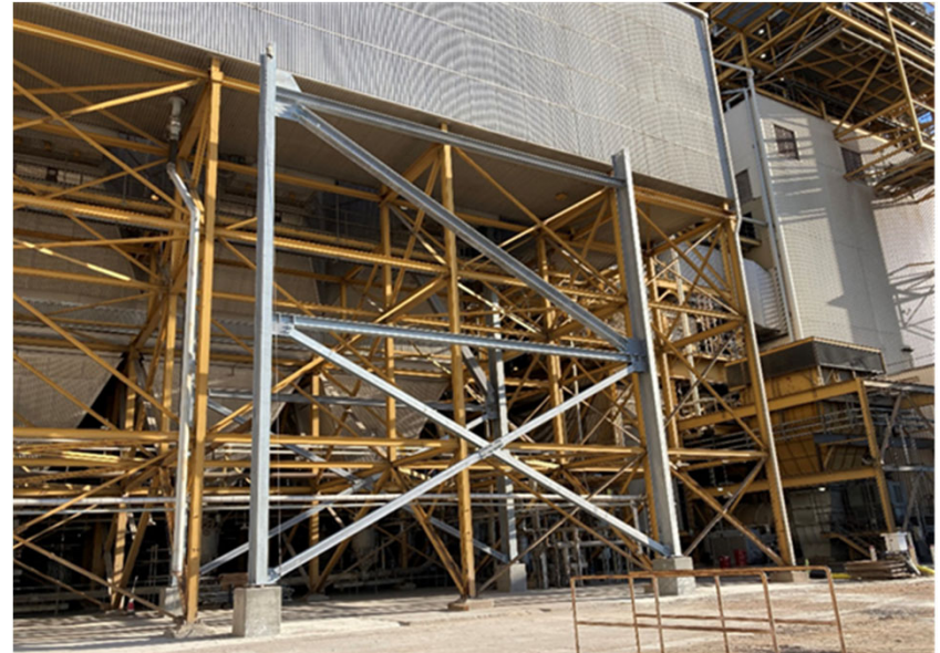
Structural Steel and Foundation
